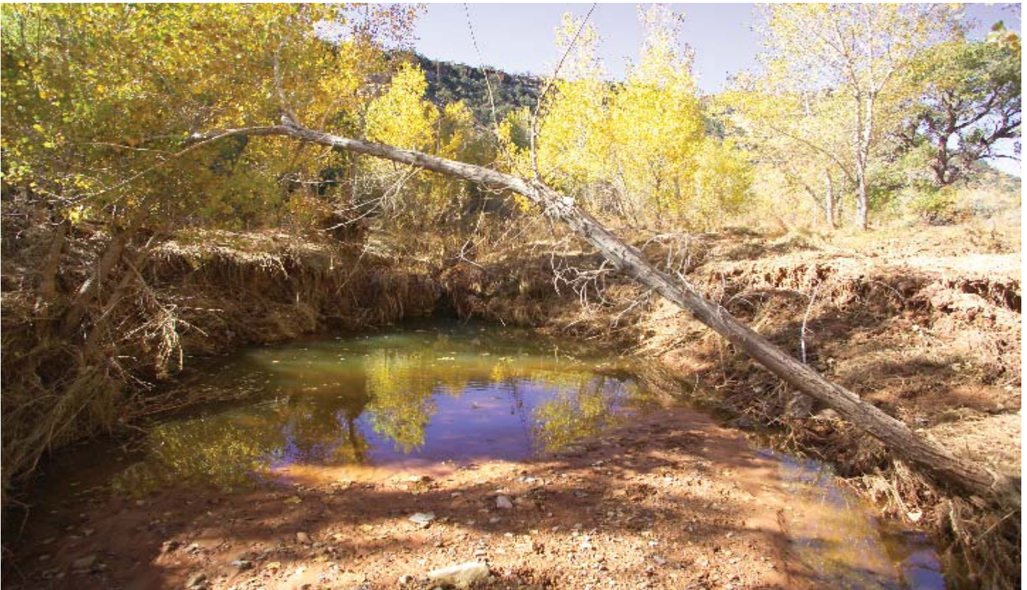
Figure 22. Additional flood damage from the tremendous energy of the flow that was augmented by the 4-wheel drive route over which much of the water flowed. Arch Canyon, San Juan County, Utah.
