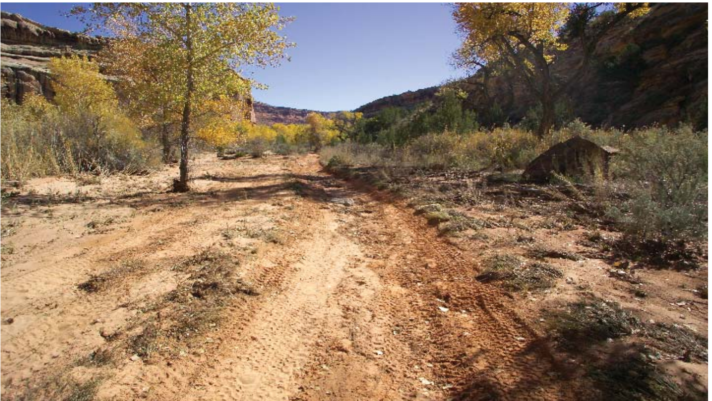
Figure 5b. Repeat photo of Figure 5a, taken in October, 2006. Flood waters jumped onto the 4-wheel drive route and caused much soil and bank erosion, and elimination of vegetation. Arch Canyon, San Juan County, Utah.
