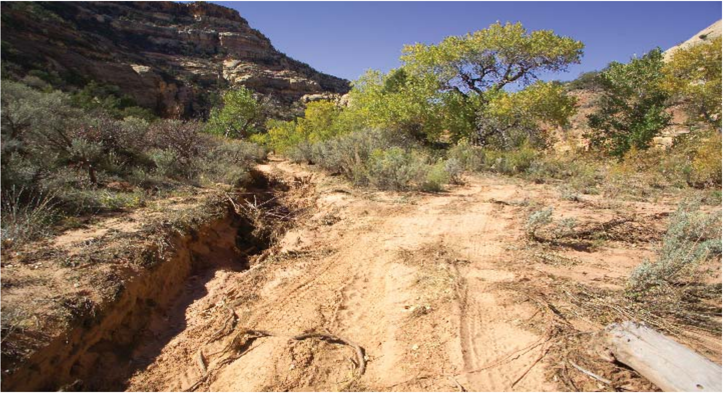
Figure 21. Photo taken in October, 2006. This is flood damage caused by water flowing down the 4-wheel drive route. The route has recently been diverted around the gully. Arch Canyon, San Juan County, Utah.
