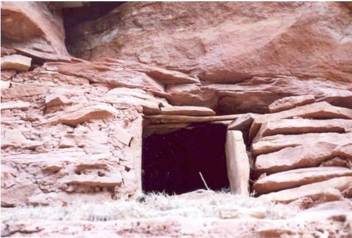
Figure 6: Close-up view of pole, stone and adobe construction at 42Sa5221, Feature B.
