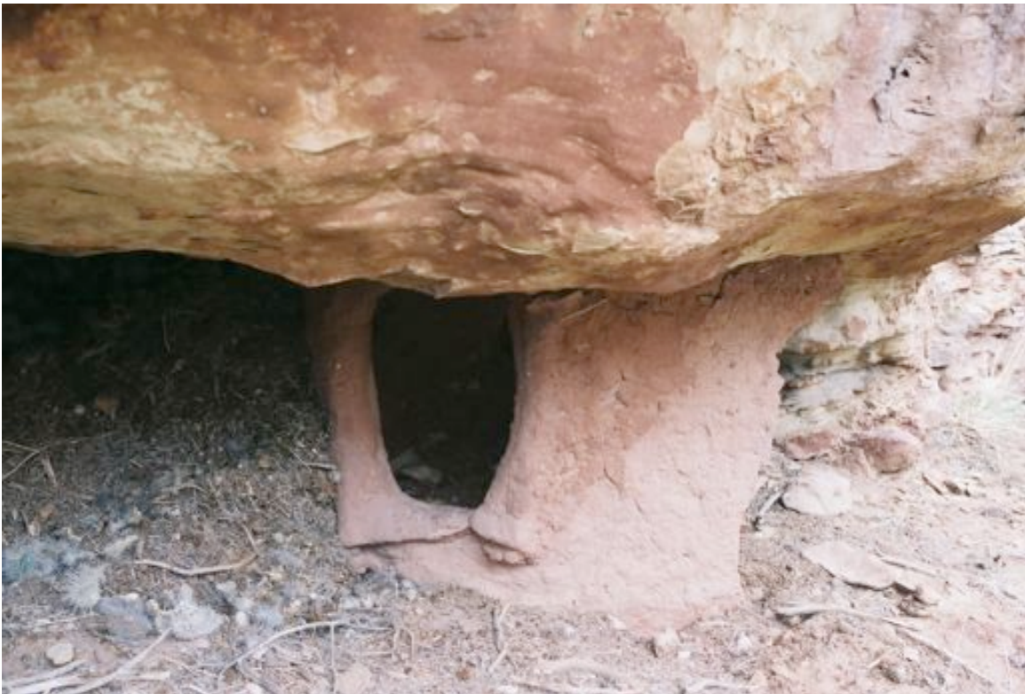
Figure 9: View of 42Sa26871, well preserved granary next to Arch Canyon vehicle access route.
